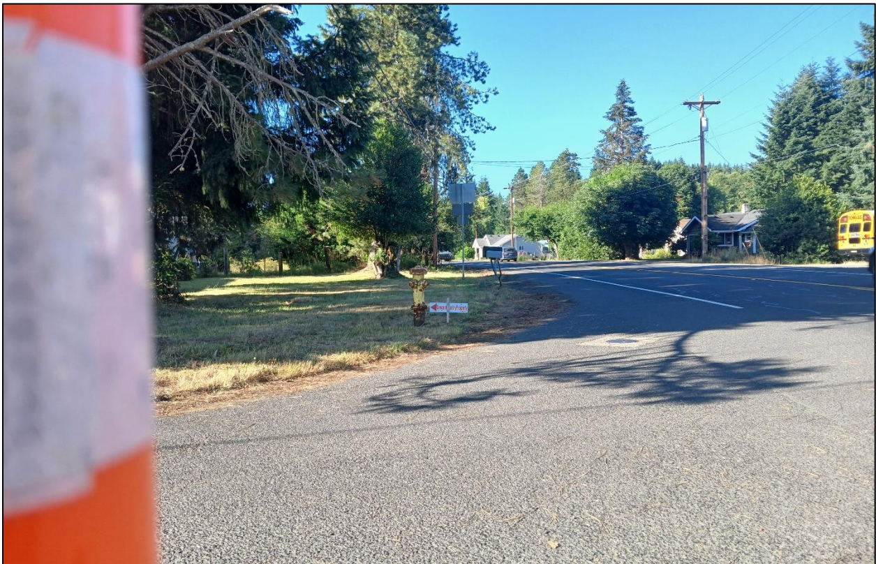
E Knott Street Looking Left (South) along Nehalem Highway (OR 47) – Available Sight Distance, 320 ft
