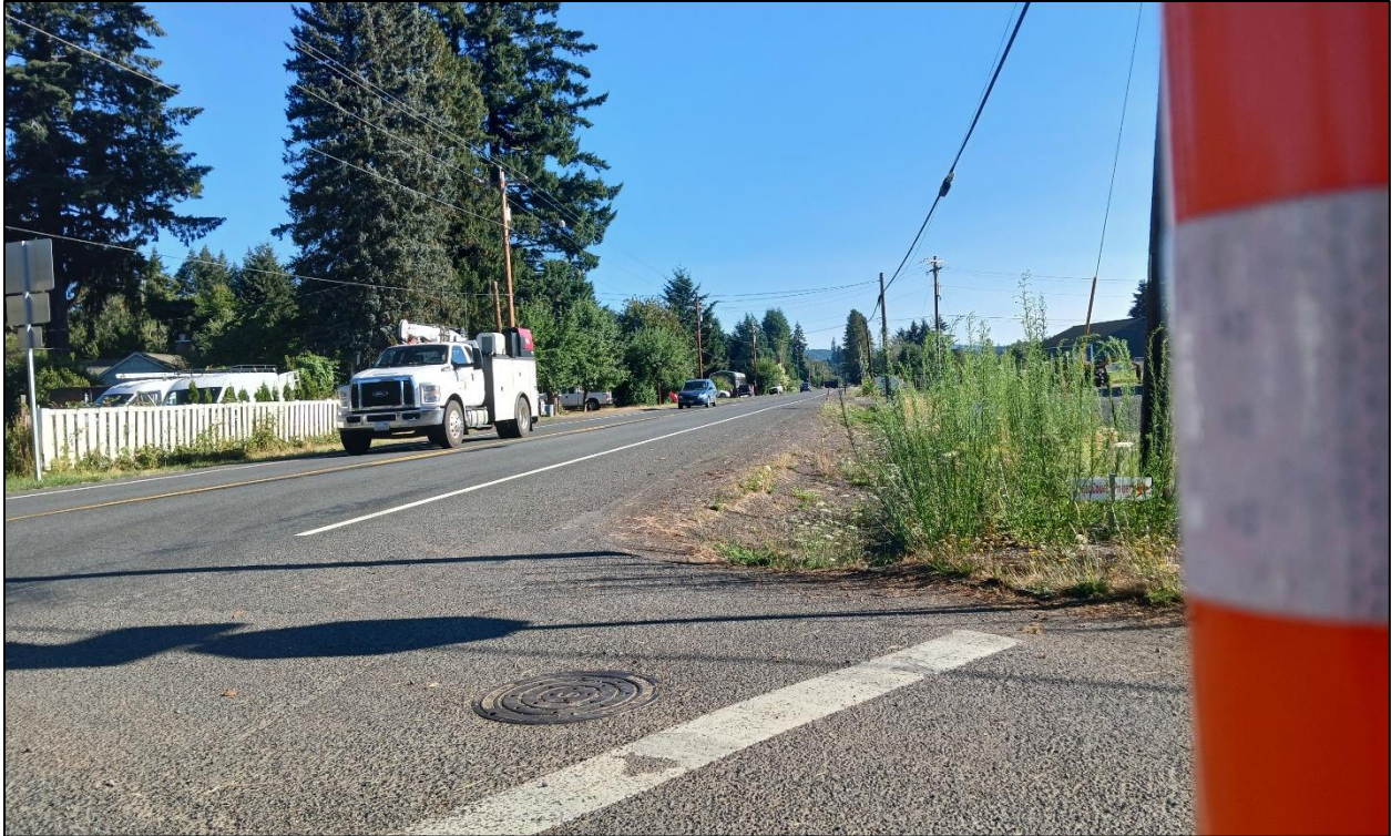
E Knott Street Looking Right (North) along Nehalem Highway (OR 47) – 1,000 ft < ISD
